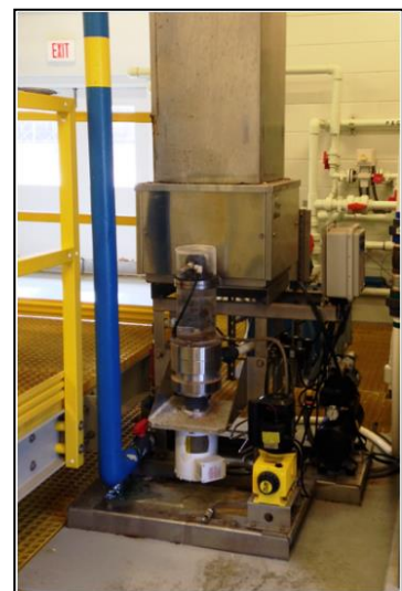
Polyblend® DP 800 Installation at Dixon, IL
